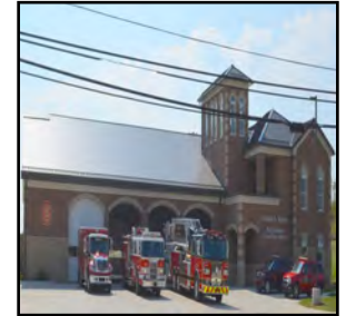
Central Fire Station
